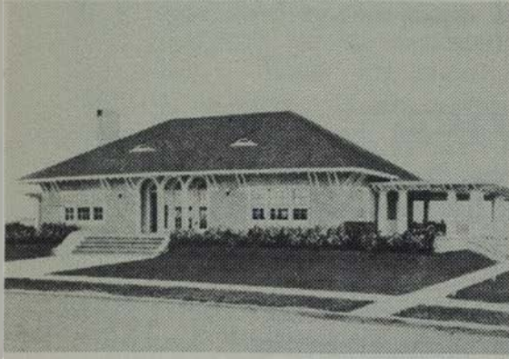
INLET TERRACE CLUB Date: 1917
